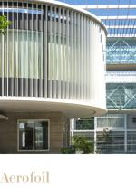
Aerofoil solar shading system is an advanced technology aiming to serve energy saving in modern buildings. These profiles can be fixed or automized to enable the residents to rotate the louvres. This allows them to alter the amount of sunlight depending on the me of day.
